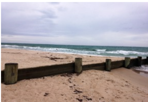
Most westerly groyne has build up of sand on western side and depletion on eastern side 1 st December 2019
